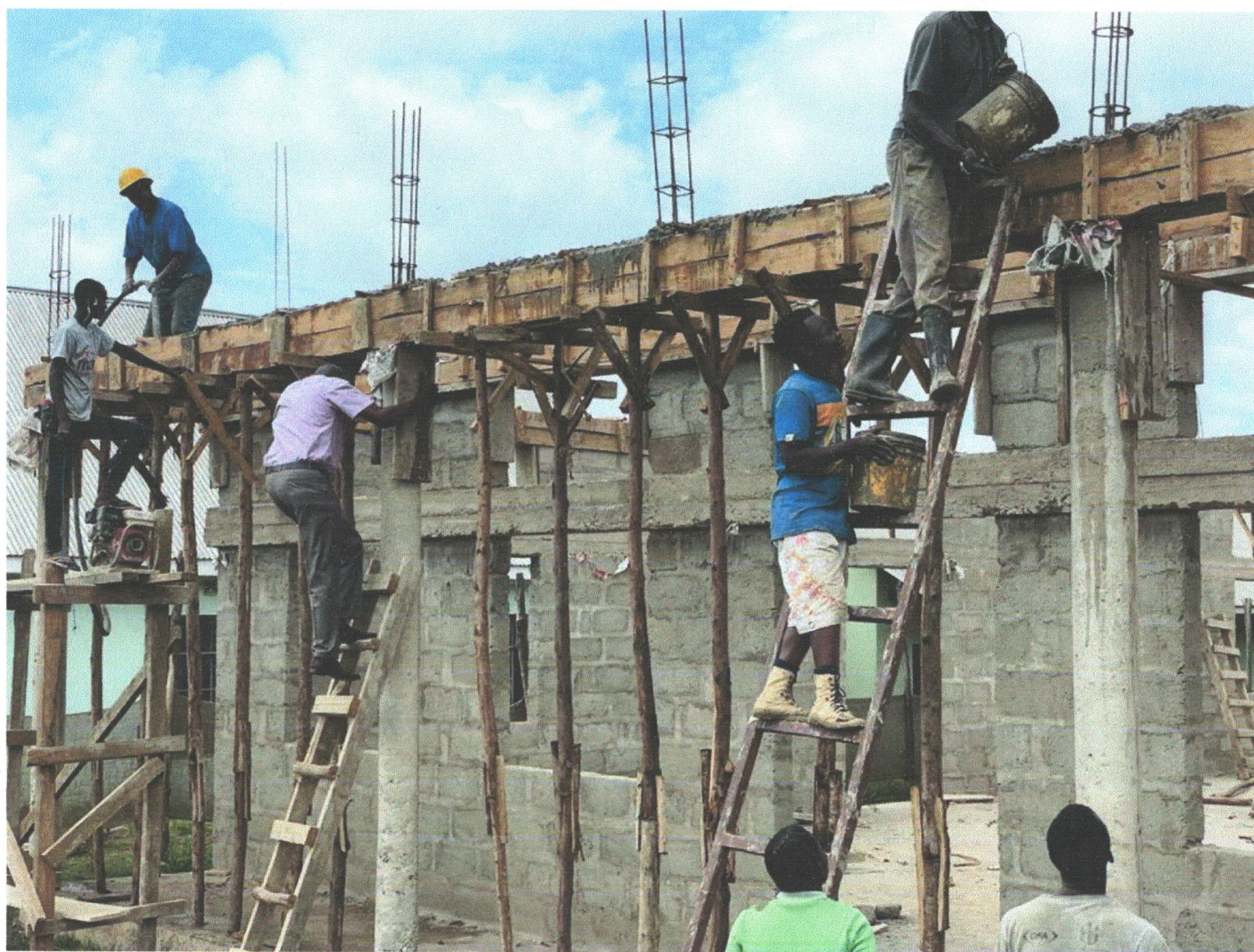
Second beam casting
